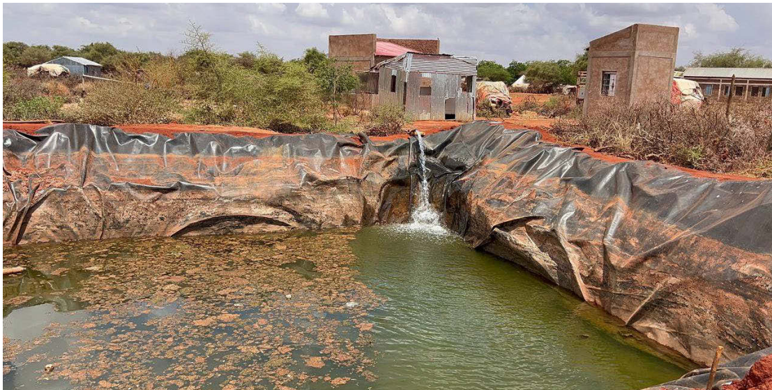
FIGURE 4: WATER FROM A DEEP BOREHOLE IN GESHAMO IS PUMPED INTO AN OPEN POND FOR COOLING
