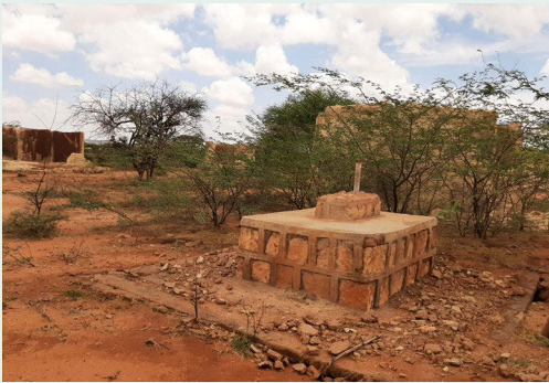
Destroyed borehole infrastructure
